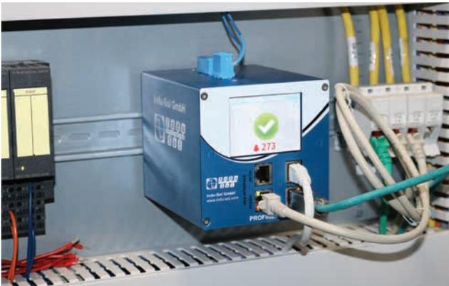
„Silent monitor” in the control cabinet: The PROFIBUS INspektor NT shows the current network overall status on the display and supplies initial diagnosis notifications.
